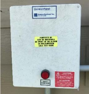
If your City-owned STEP system sounds an alarm, you can silence it by pushing the RED button on the STEP system control panel and then immediately call the Wastewater Division at the number located on your box, (406) 523-4886. We have collection staff ready to respond at any time, day or night, including weekends and holidays.
