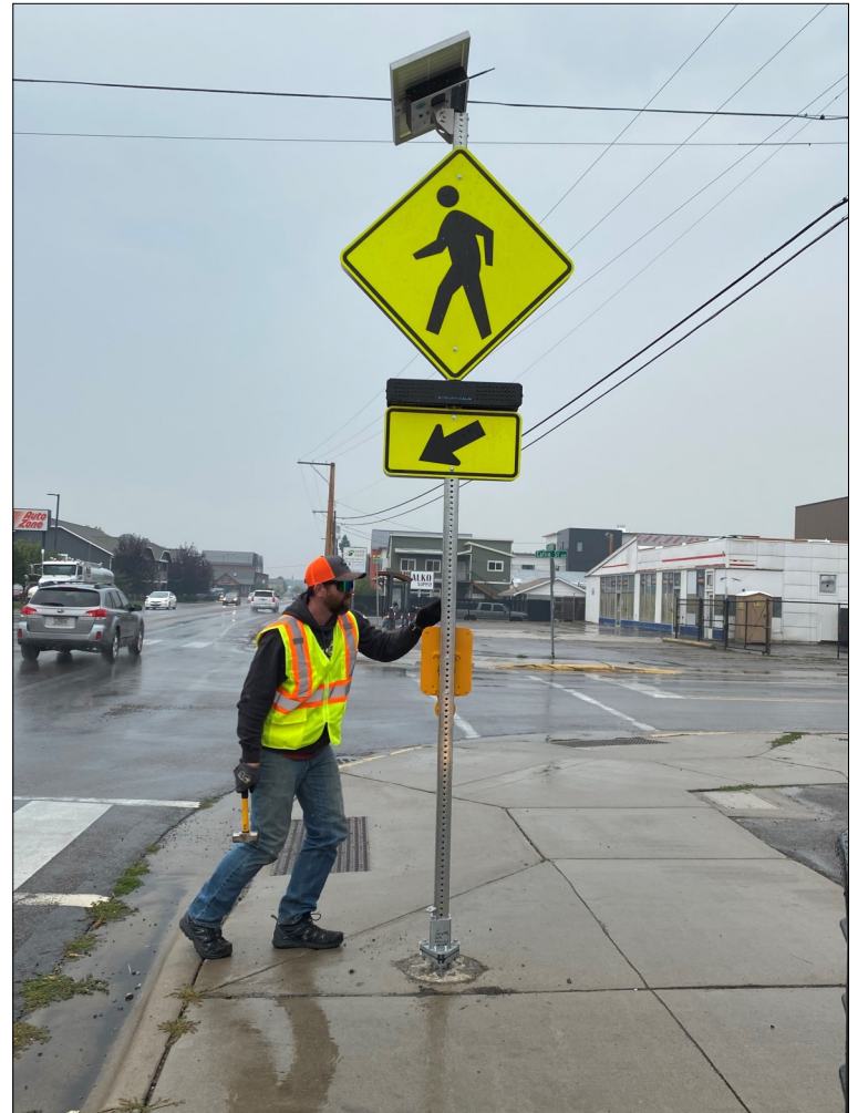
Above: Rectangular rapid-flashing beacons (RRFBs) are pedestrian-activated safety features that are installed at locations where drivers may need enhanced notification that people are crossing the street.
