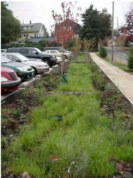
Figure 5-8: A vegetated swale filters stormwater runoff from a parking lot
