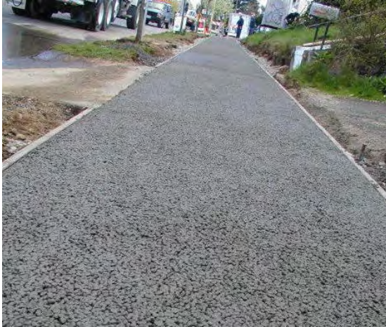
Figure 5-7: A pervious concrete sidewalk
