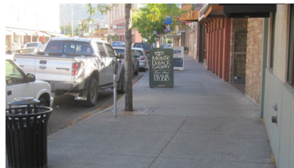
Substandard sidewalk further compromised by overly large and incorrectly placed signs
