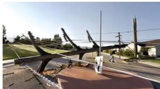
Several poles in the Upper Linda Vista neighborhood snapped off during the storm. Source: Missoulain
