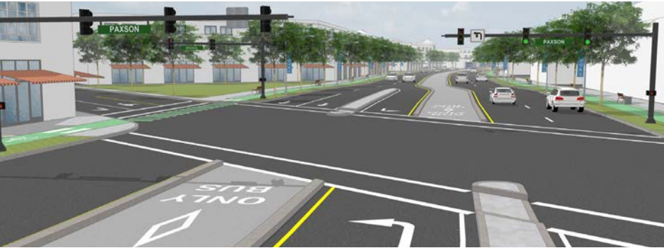
Signalized left turns at key locations permit U-turns and provide safe crossing of the bus lane and access to destinations on the opposite side of Brooks Street.
