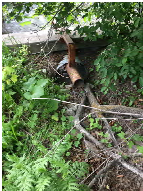
Photo 32. SNA-1570 clogged channel (6/2/2020)
