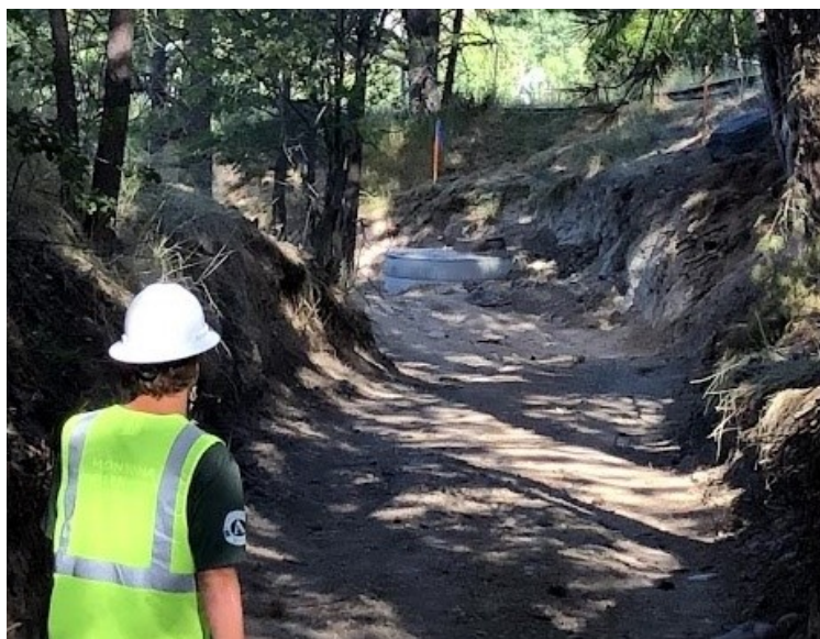
Gharrett Drainage following StormGate installation.
