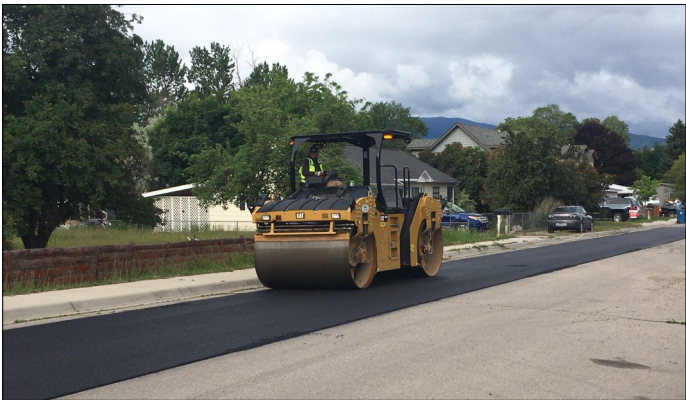
A steel wheel roller is used to compact newly applied asphalt.
