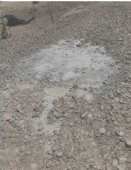
Onsite at a SWPPP inspection, concrete washout into open gravel. These SWPPP inspections are valuable opportunities to educate our building community on the dangers of water pollution created by insufficient BMP's.
