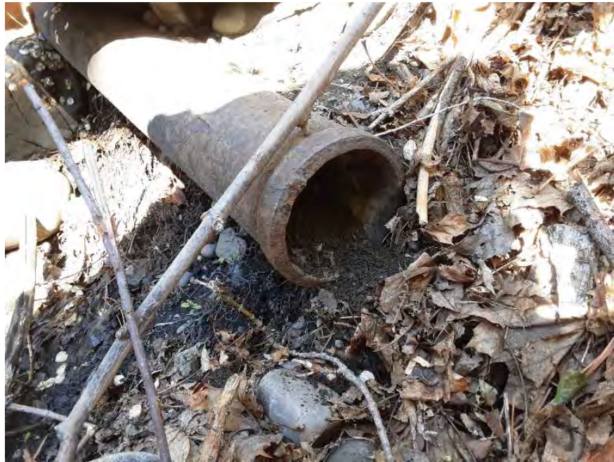
Photo 38. Outfall Pipe UNK-27 partially filled with sediment (6/2/2020)
