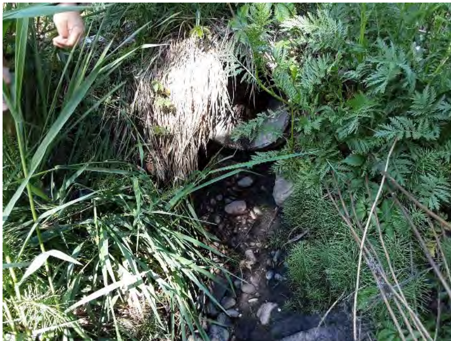
Photo 37. Outfall Pipe SNA-1534 with excessive vegetation (6/2/2020)
