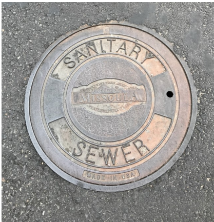
Sewer system manhole lid.
