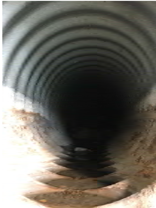
Photo 36. SNA-1568 Minor Corrosion and stains inside Out Pipe (6/2/2020)
