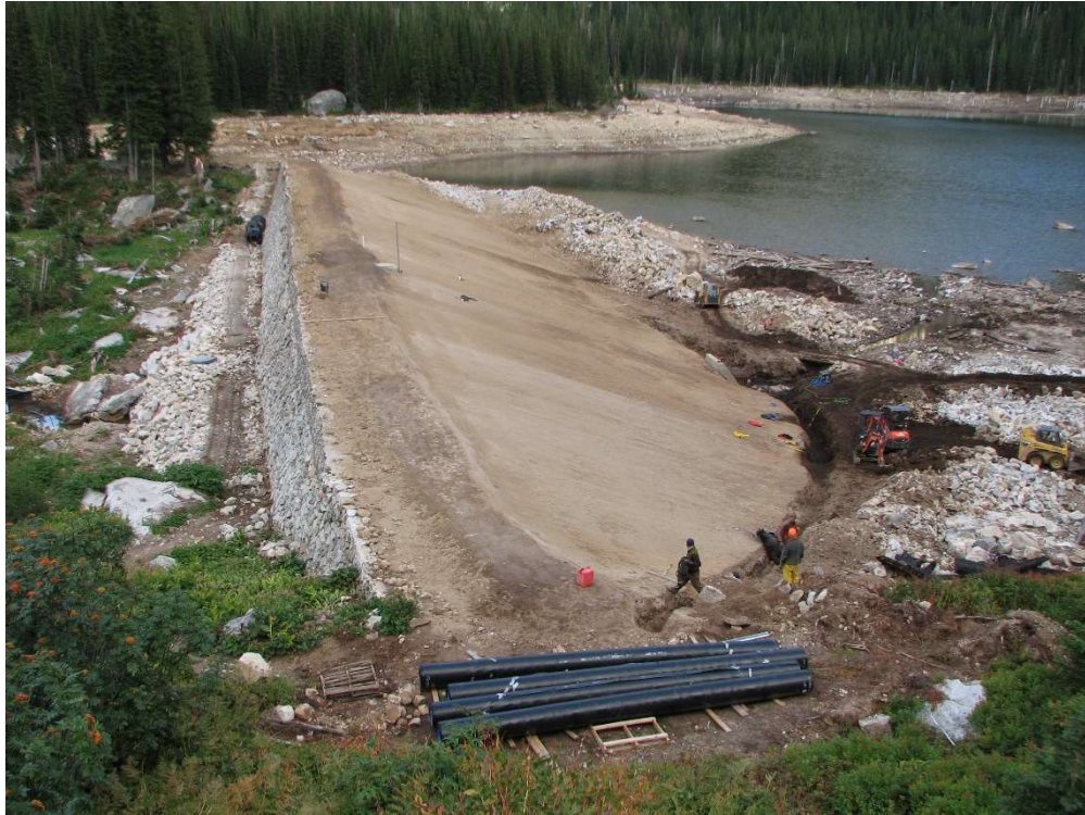
Figure 9-5. Mill Lake Dam, Geomembrane Liner Installation
