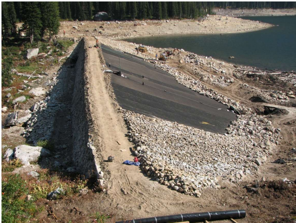
Figure 9-6. Mill Lake Dam, Geomembrane Liner and Riprap Installation
