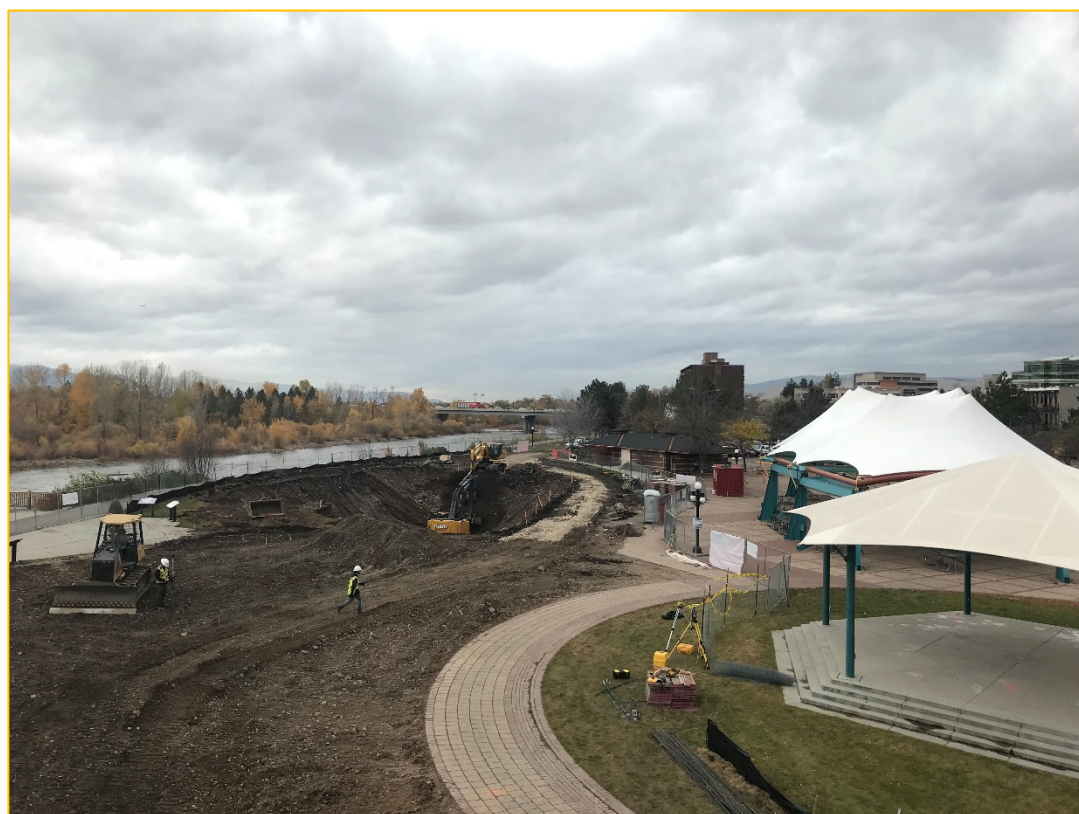
Left: The Stormwater Utility recently began a project in Caras Park to install an infiltration gallery that will collect the first one-half inch of stormwater runoff from the downtown area to prevent dissolved pollutants from entering the Clark Fork River.
