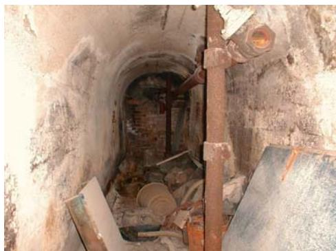
system also remain under sidewalks and park area adjacent to the Bank building. Although portions of the tunnel system have been cleaned, some of the tunnels are still lined with asbestos. The structural integrity of tunnels and some piping is beginning to deteriorate to a point that they will require focused attention in coming years. Additional relics of the area's historic industrial past have been found recently in the form of a honeycomb of large concrete
