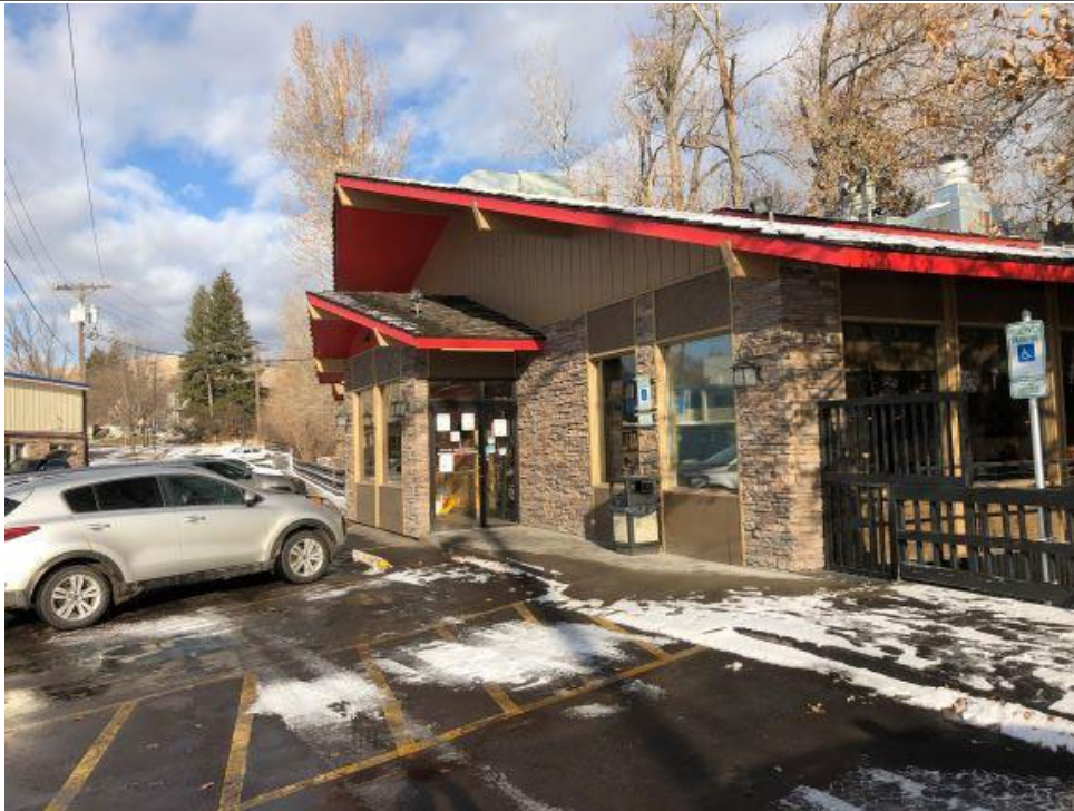
Photo One Caption West Side Main Building Entrance
