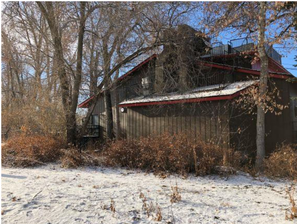
Photo Two Caption East Side of Building with Equipment Location in Cropout
