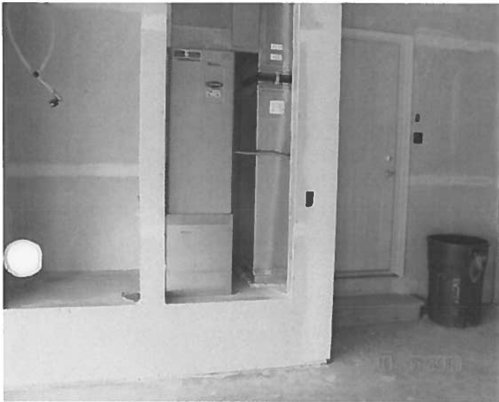
Furnace on elevated platform in garage
