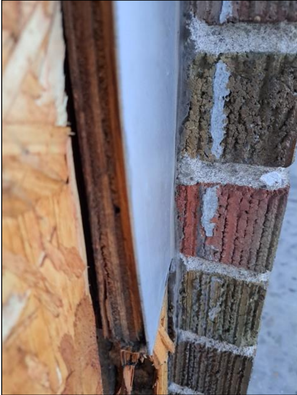
Plywood used to frame the pony wall.
