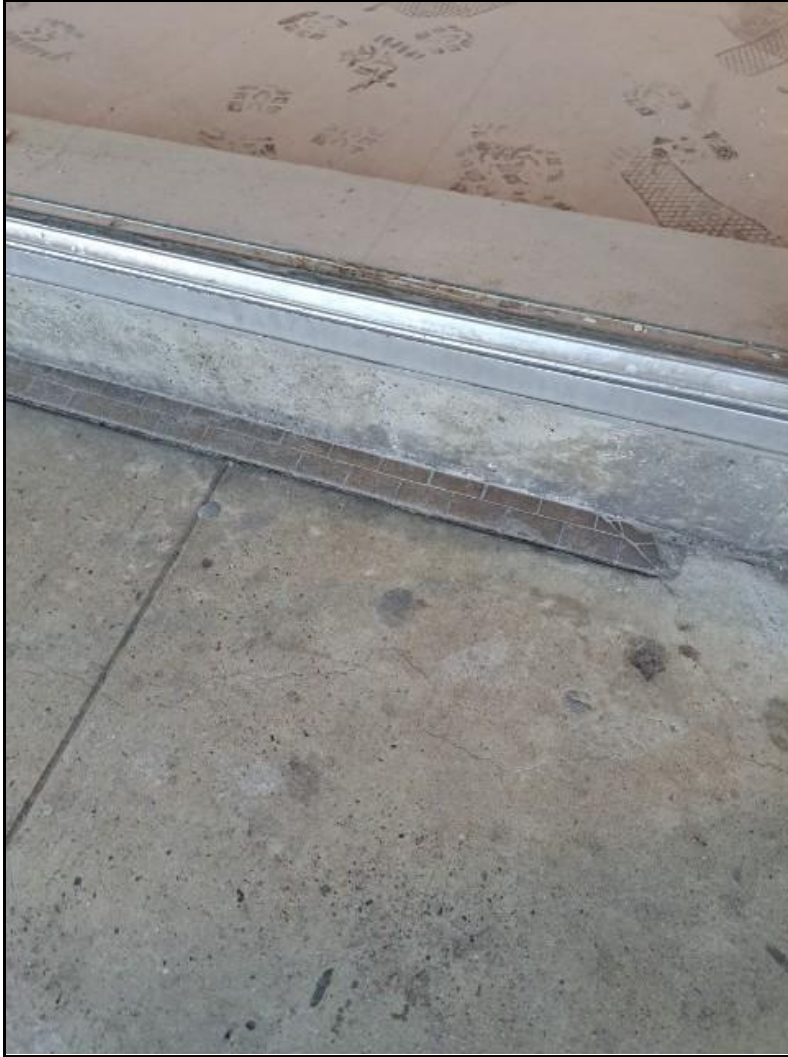
Non-historic concrete window base of retail glass in corner suite. Proposed for removal. Note the tile below the concrete demonstrates it is non-original.
