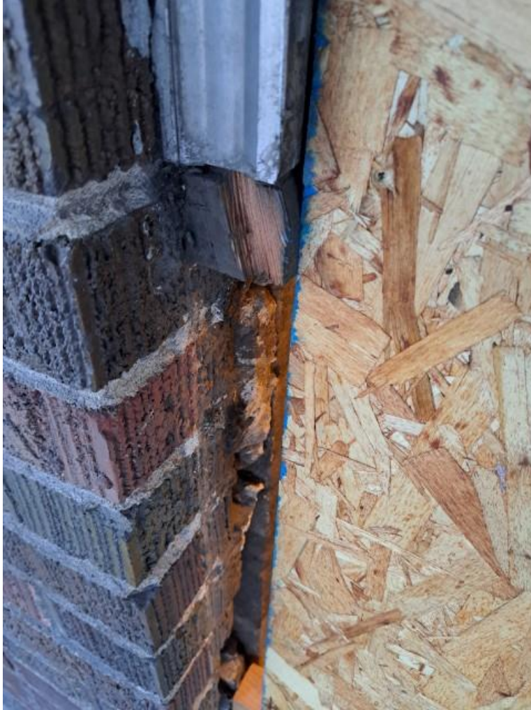
View of where the trim and lumber was cut to accommodate the addition of the pony wall.
