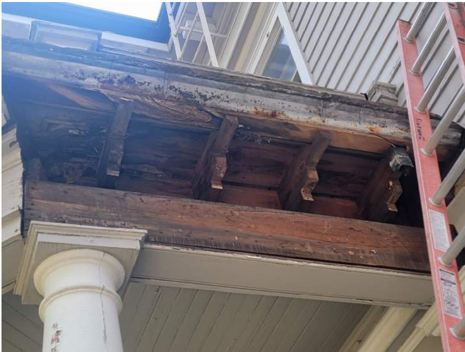
Photo #5: Rafters cantilevering past end beam – dry rot. End Beam bears totally on column.
