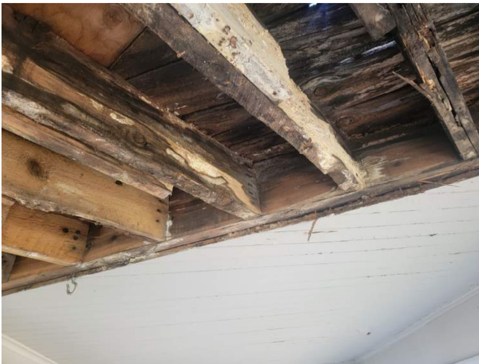
Photo #3: Dry Rot prevalent throughout the 2x rafters and diagonal beam
