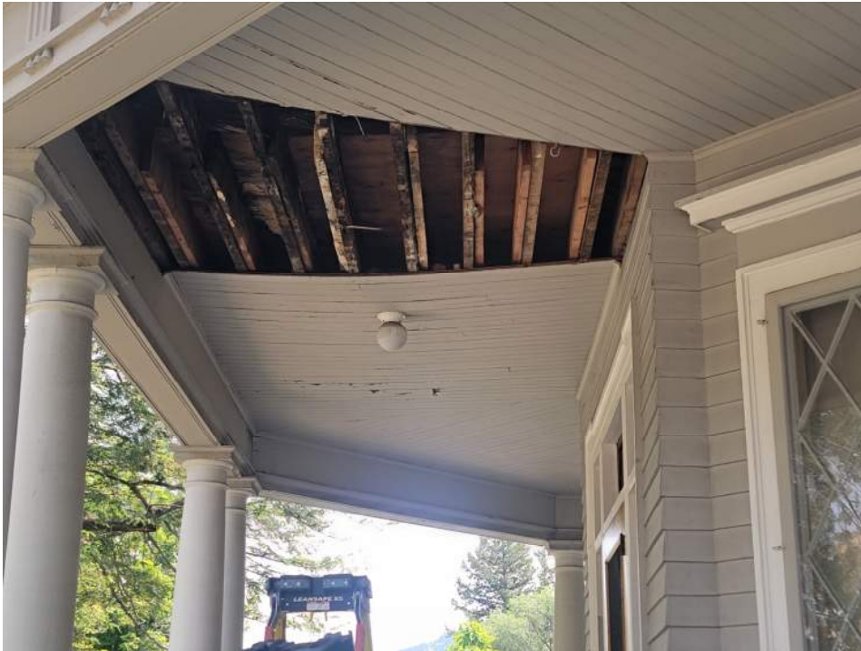
Photo #2: Area that was sagging and has been partially opened up from below
