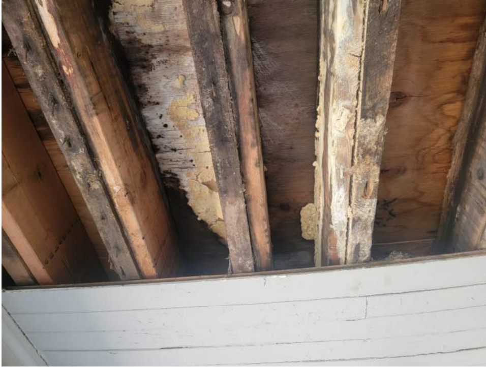
Photo #4: Signs of past repair work from above with doubled members and plywood sheathing
