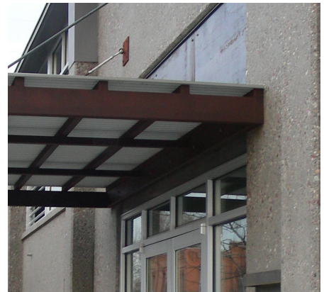
Conglomerate concrete and metal detailing
