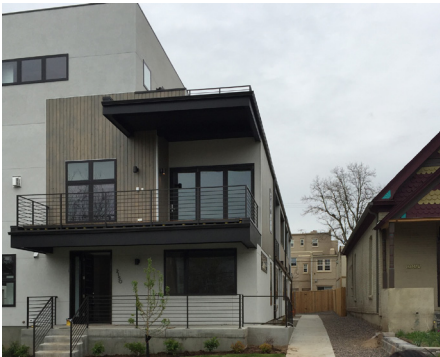
The multifamily building steps down to single-family residential building, providing a compatible transition in building height.
