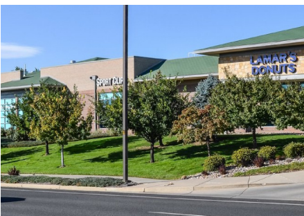
Landscaped edge/buildings set back (buildings are also allowed closer to the street)
