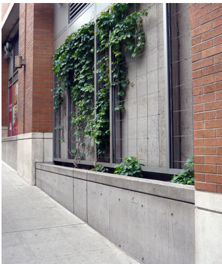
Vertical wall landscaping
