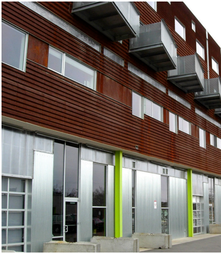
This building reflects a connection to the environment in its design by incorporating wood siding.
