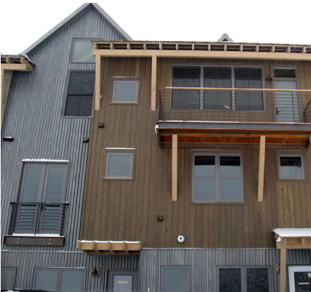
Wood siding with corrugated metal
