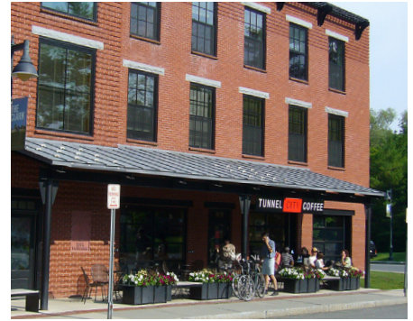
Parking behind building
