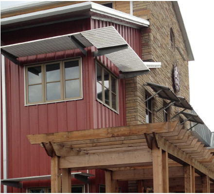
Stone siding and wood pergola with metal siding
