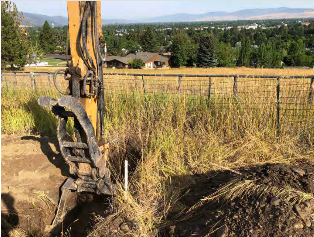
Description: TP-02 Piezometer being backfilled. View is to the northwest.
