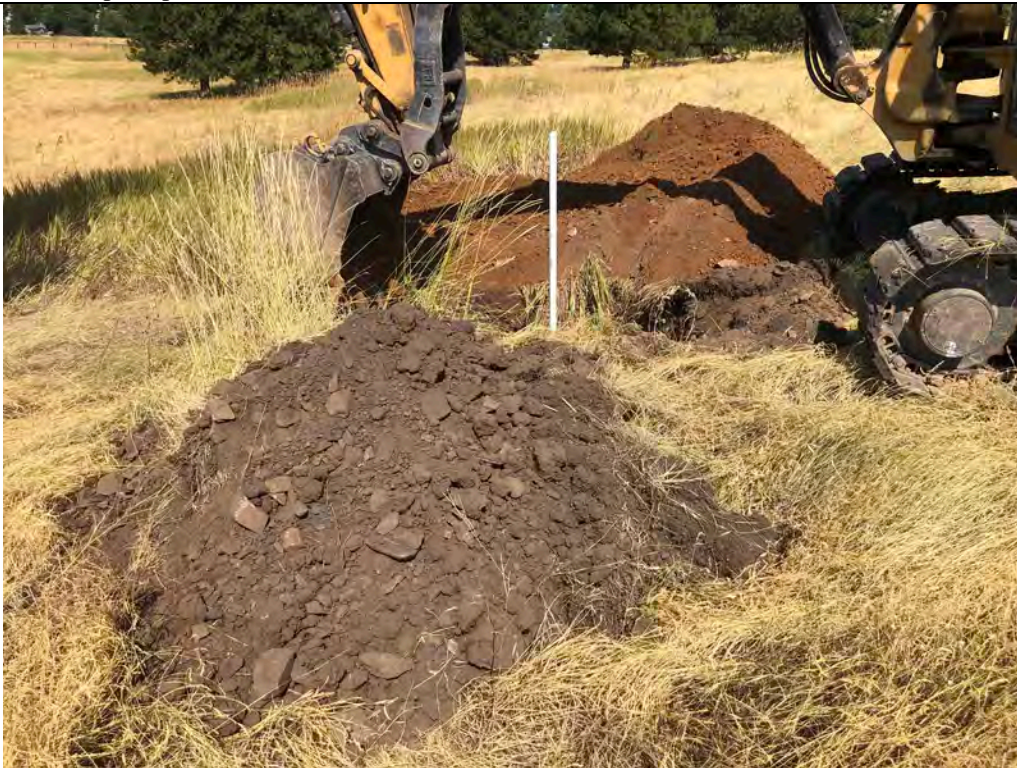
Description: TP-07 Piezometer being backfilled. View is to the west.
