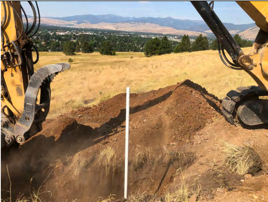
Description: TP-10 Piezometer being backfilled. View is to the north.
