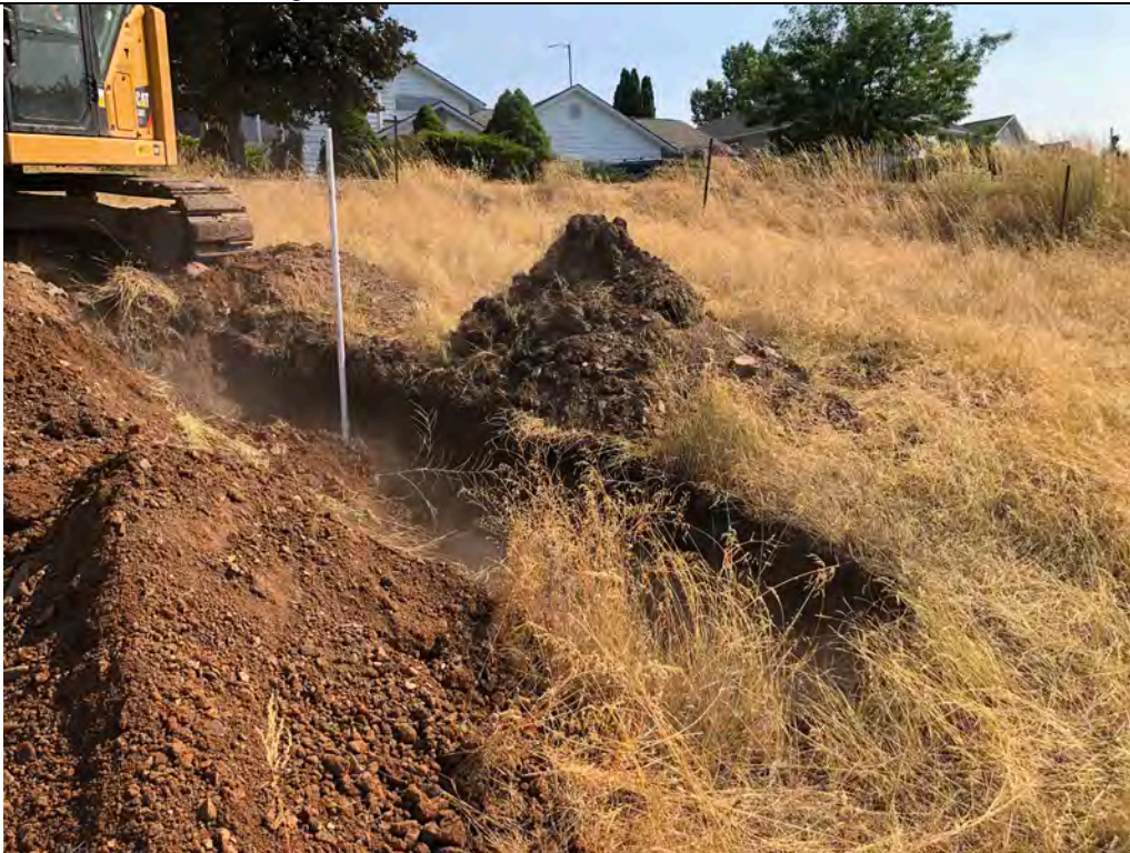
Description: TP-10 Piezometer being backfilled. View is to the south.
