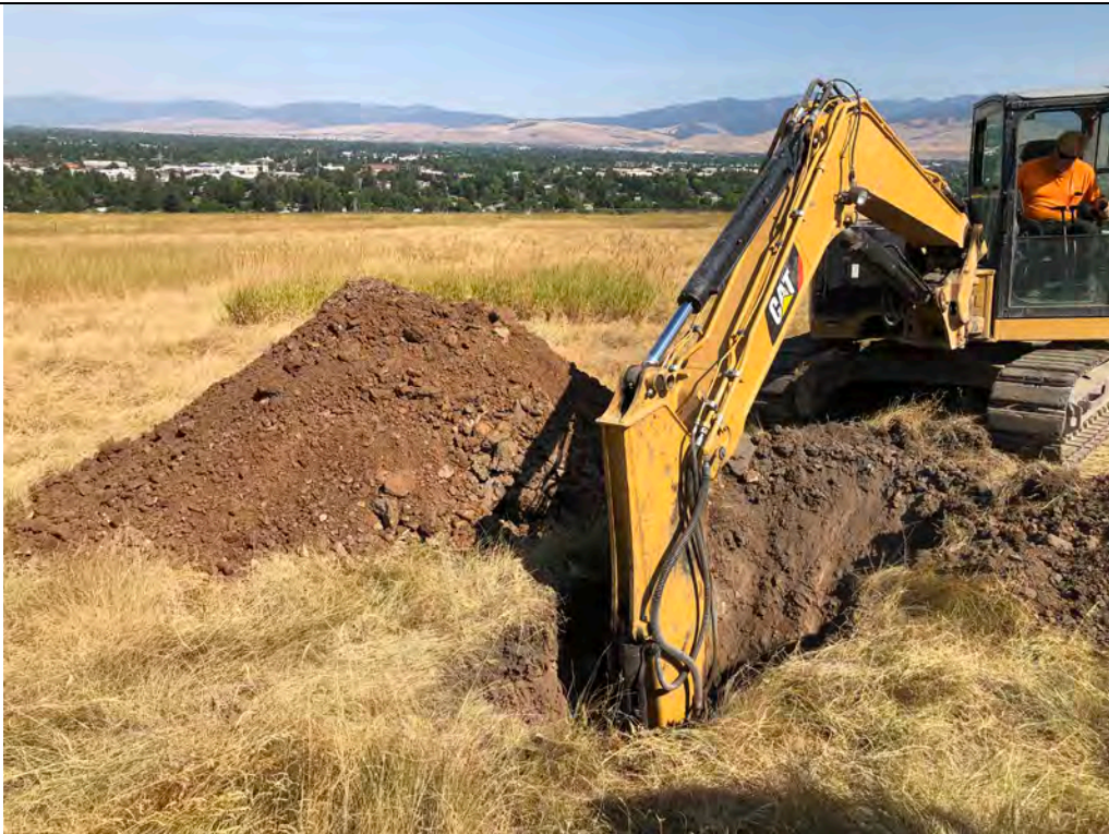
Description: TP-06 Location. View is to the north. Cone penetrometer (not shown) was pushed 3.25 inches at the ground surface under a 320 psi loading.
