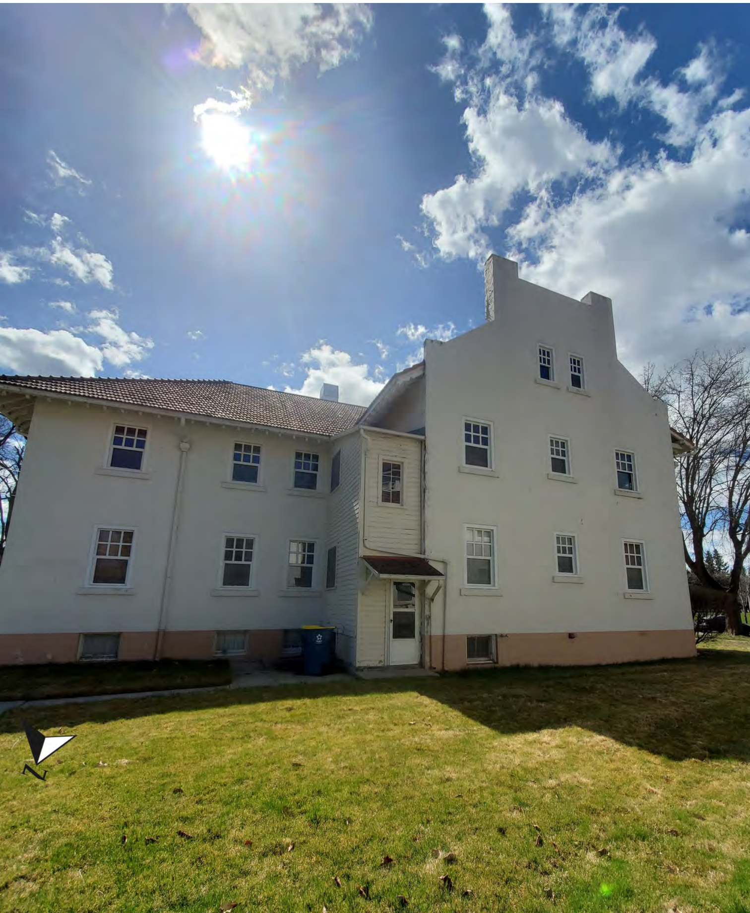
NORTH PARAPET WALL
