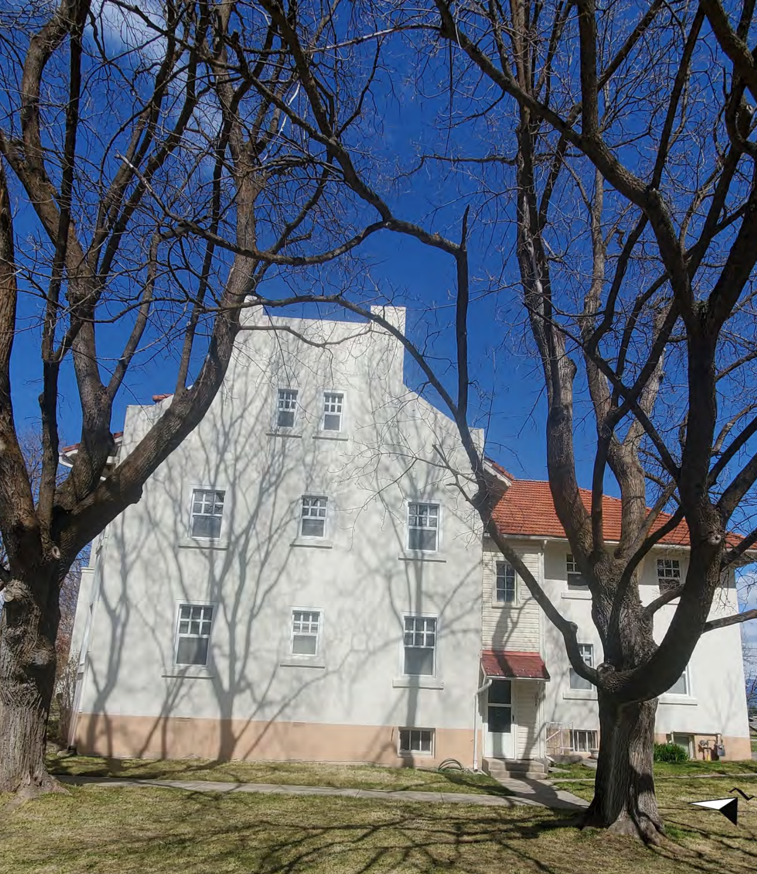
SOUTHSIDE PARAPET WALL
