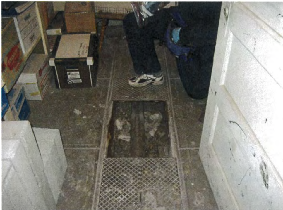
Photo 19: Underground pipe in basement (storage room 09) with debris.
