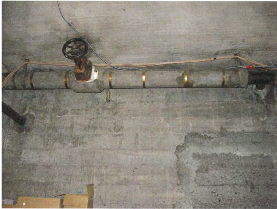
Photo 15: Piping insulation in basement.
