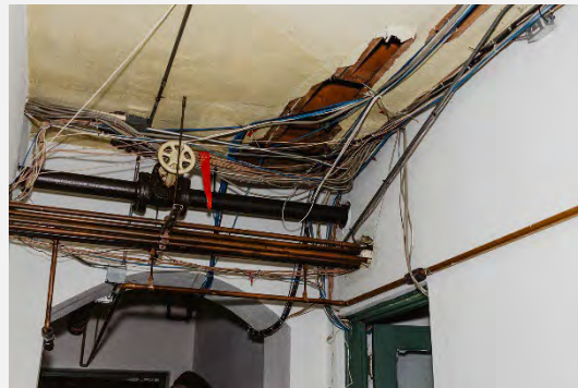
Questionable wiring, failed finishes
