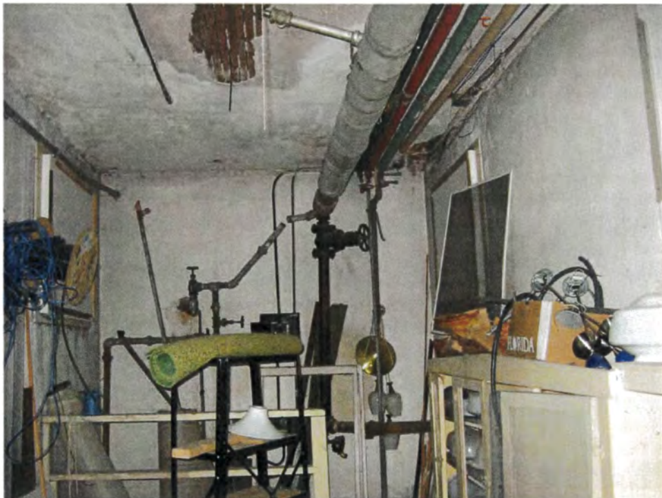
Photo 20: Exposed insulation in basement (storage room 03).
