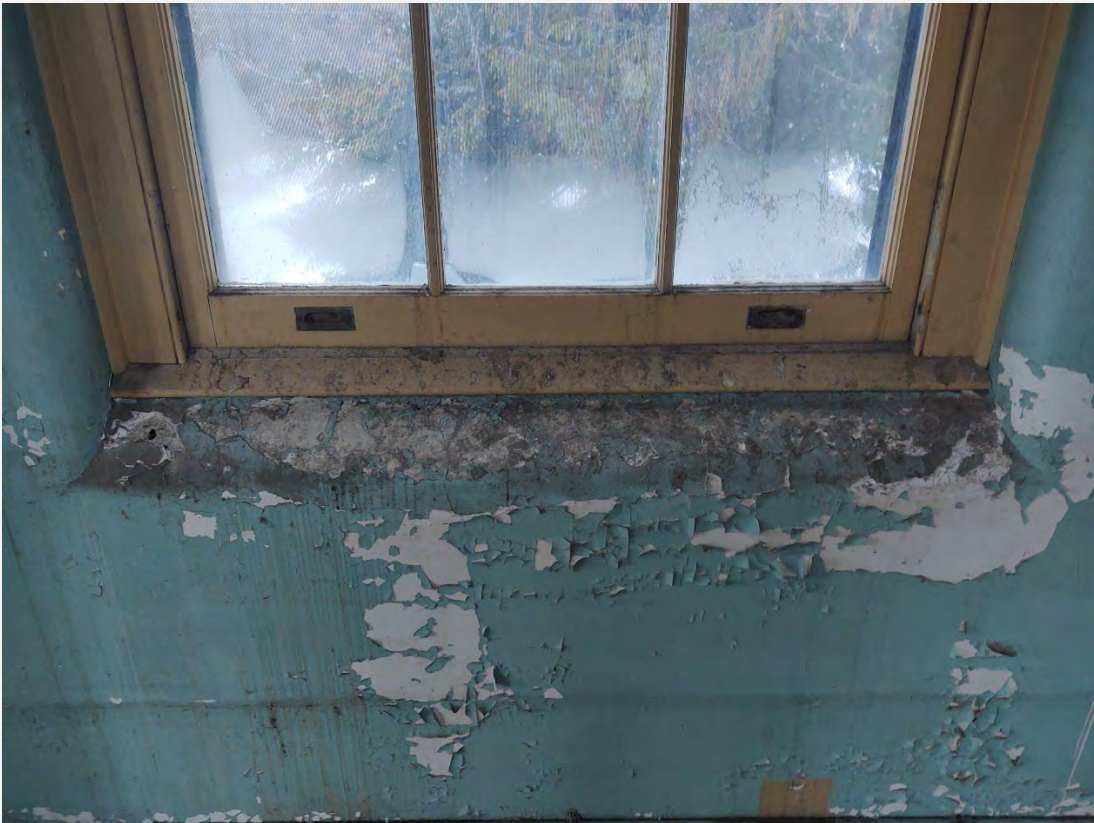
Water Damage from single pane glazing. Window painted shut with Lead based paint
