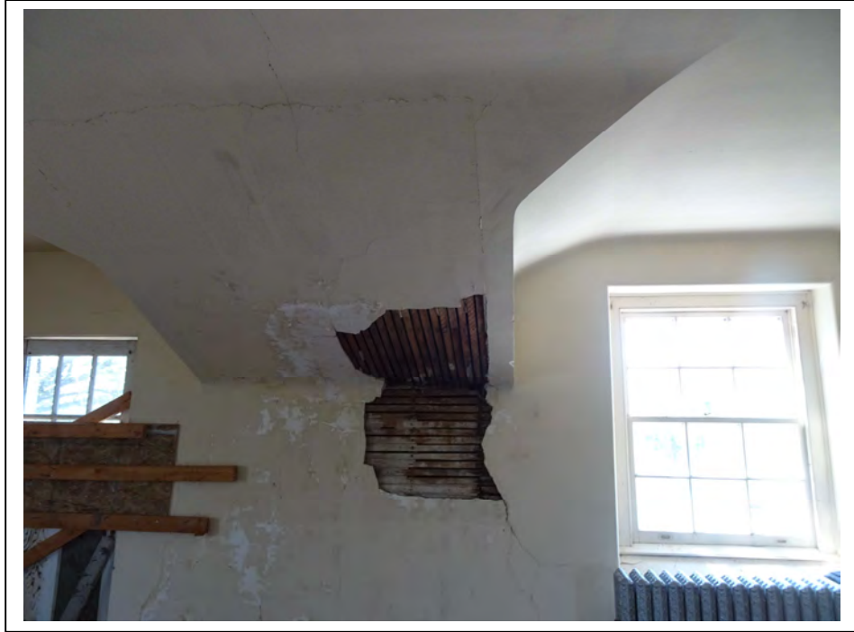
View of interior showing damage and deterioration to wall & ceiling
