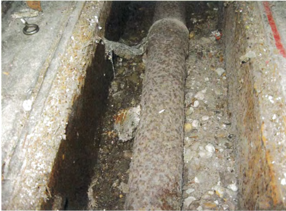
Photo 23: Subterranean pipe with debris, in basement.
