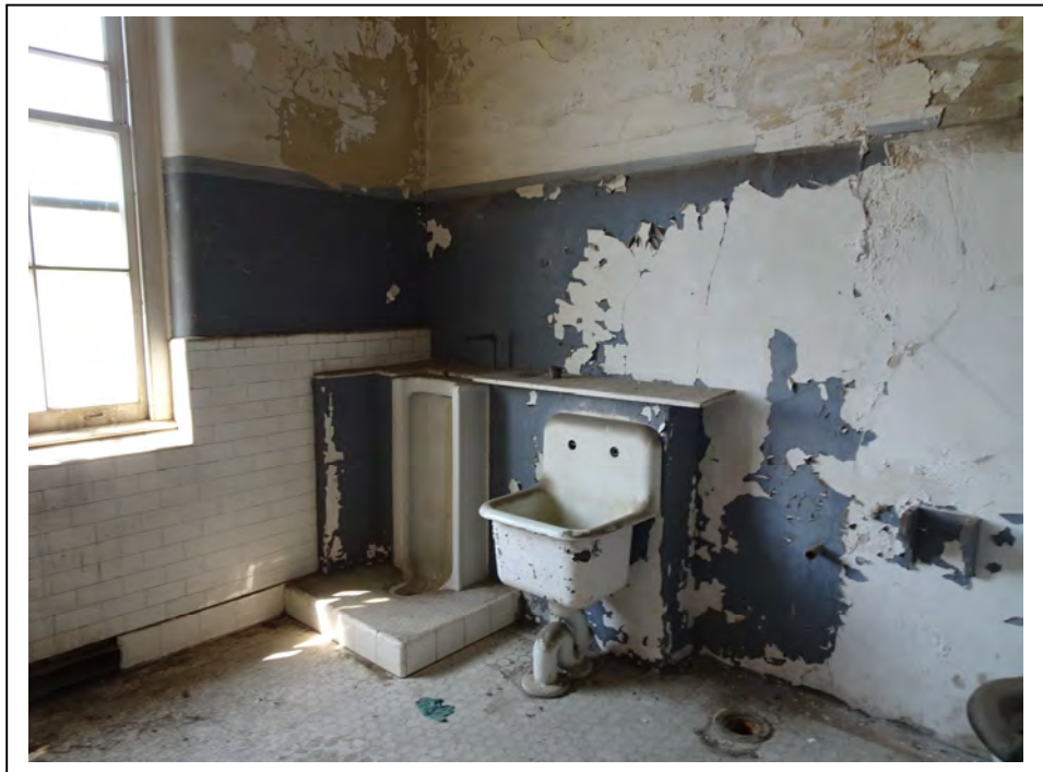
Typical view of original plumbing at several areas in the building
