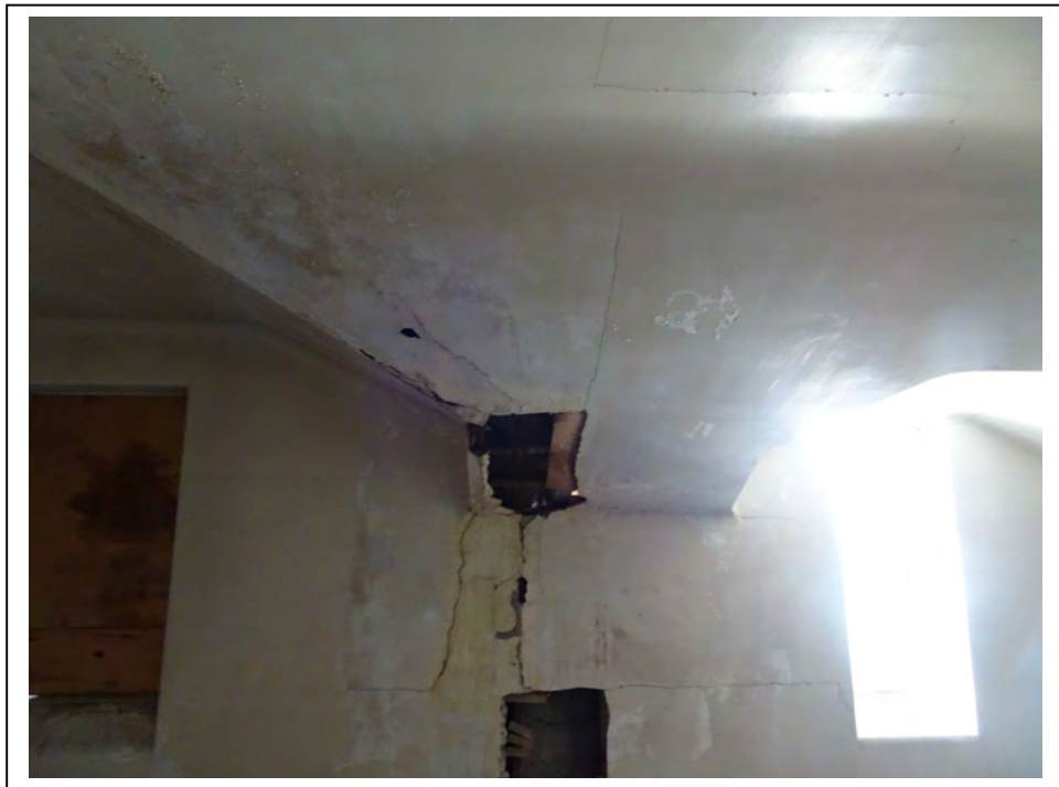
View of interior showing damage and deterioration to ceiling
