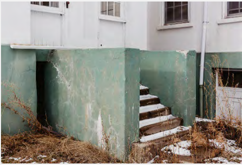
Deteriorated Concrete and Stucco
