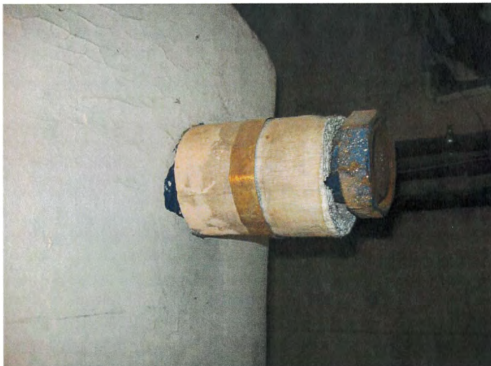
Photo 14: Insulation on small boiler in basement.
