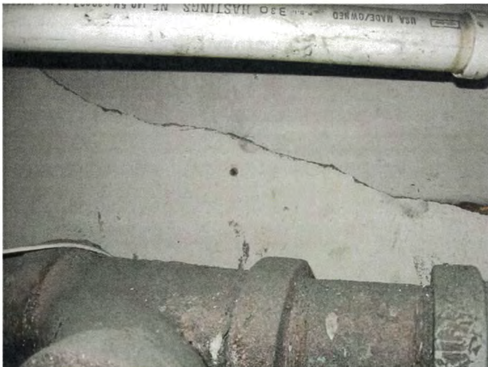
Photo 24: Transite roofing in boiler room of basement.
