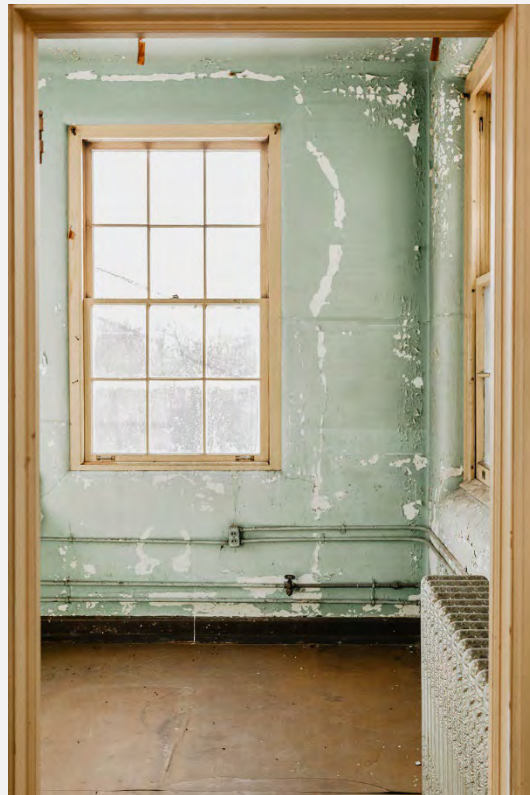
Failing Finishes due to water leaks.
