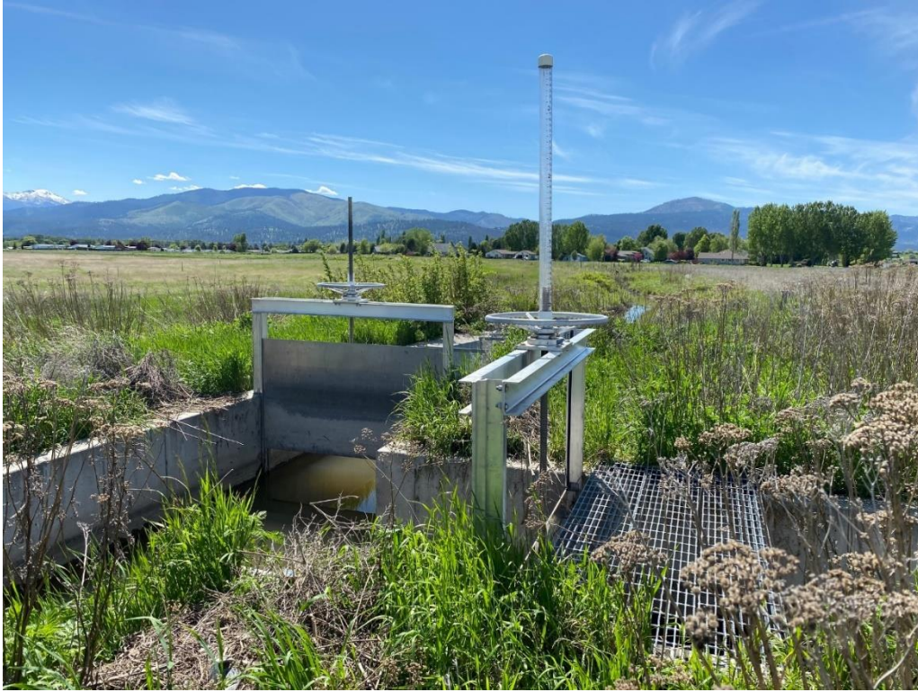
Figure 17. Newly constructed structure between George Elmer Drive and Chuckwagon Drive. View to the southwest. The headgate on the right directs flow into L2 and is a reconfiguration of the historic diversion point for L2.
