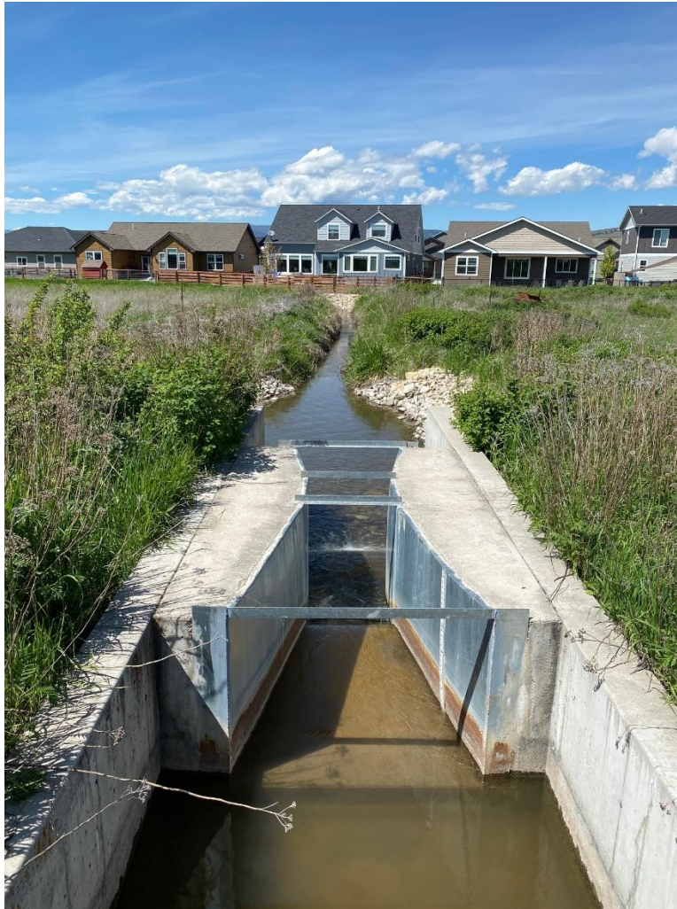
Figure 18. Newly constructed Parshall Flume at a lateral (L2) diversion point between George Elmer Drive and Chuckwagon Drive. View to the north.
