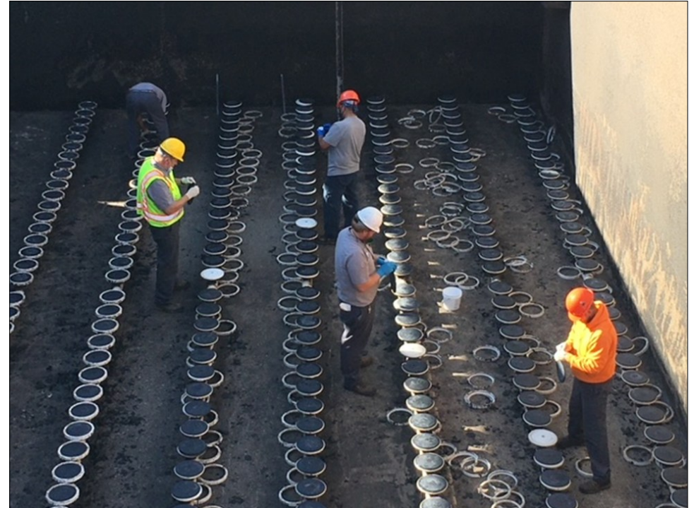
Wastewater Treatment Plant staff replace the 1,900 diffuser membranes in each of the four bioreactors about every seven years. The bioreactors are the part of the wastewater treatment process that uses microorganisms to further break down organic waste and pollutants, helping to bring water quality to Montana Department of Environmental Quality-approved levels before it is discharged to the nearby Poplar Farm or into the Clark Fork River.
