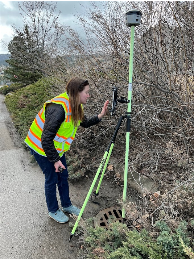
Stormwater Utility staff continue to collect Geographic Information Systems (GIS) location data for stormwater inlets and other stormwater infrastructure. This allows them to monitor the condition of the structures and develop maintenance schedules. The inlet locations are shown on a public-facing map that residents can use to report issues.
