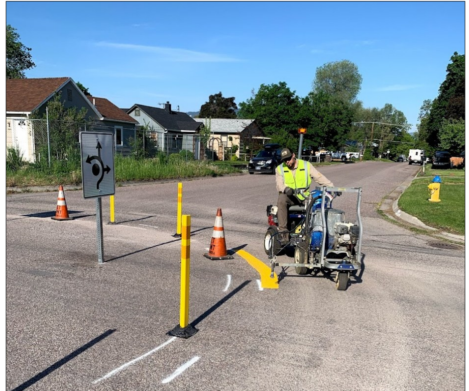
Above: Sign Shop staff install the delineators, signs, and striping on City quick-build projects. Residents can work with their neighborhood councils to paint or make other improvements to the area inside the circles.
