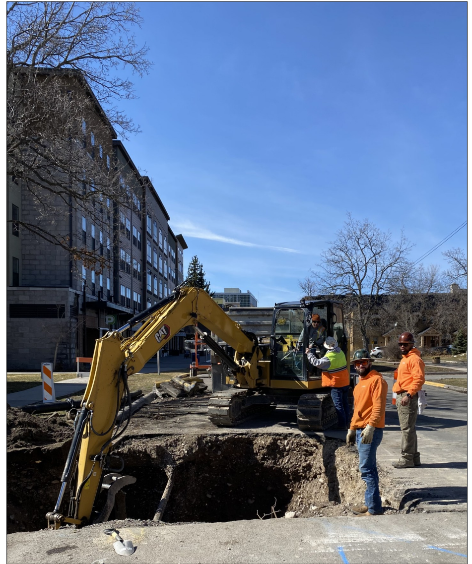
Missoula Water staff work with a contractor to replace an old fire hydrant in Downtown Missoula.
