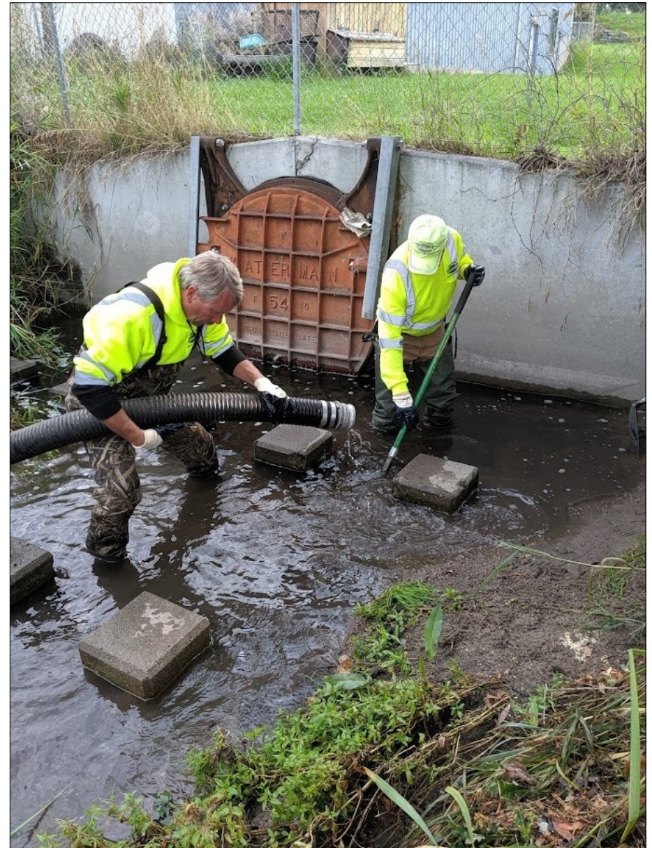
Wastewater Utility staff assist the Stormwater Utility by using a vac truck to help clean the Bitterroot Outfall area. The upcoming Bitterroot Outfall Project will improve river water quality by installing infrastructure that filters out sediment from the stormwater before it reaches the river. The project will also provide better access to perform maintenance work.
