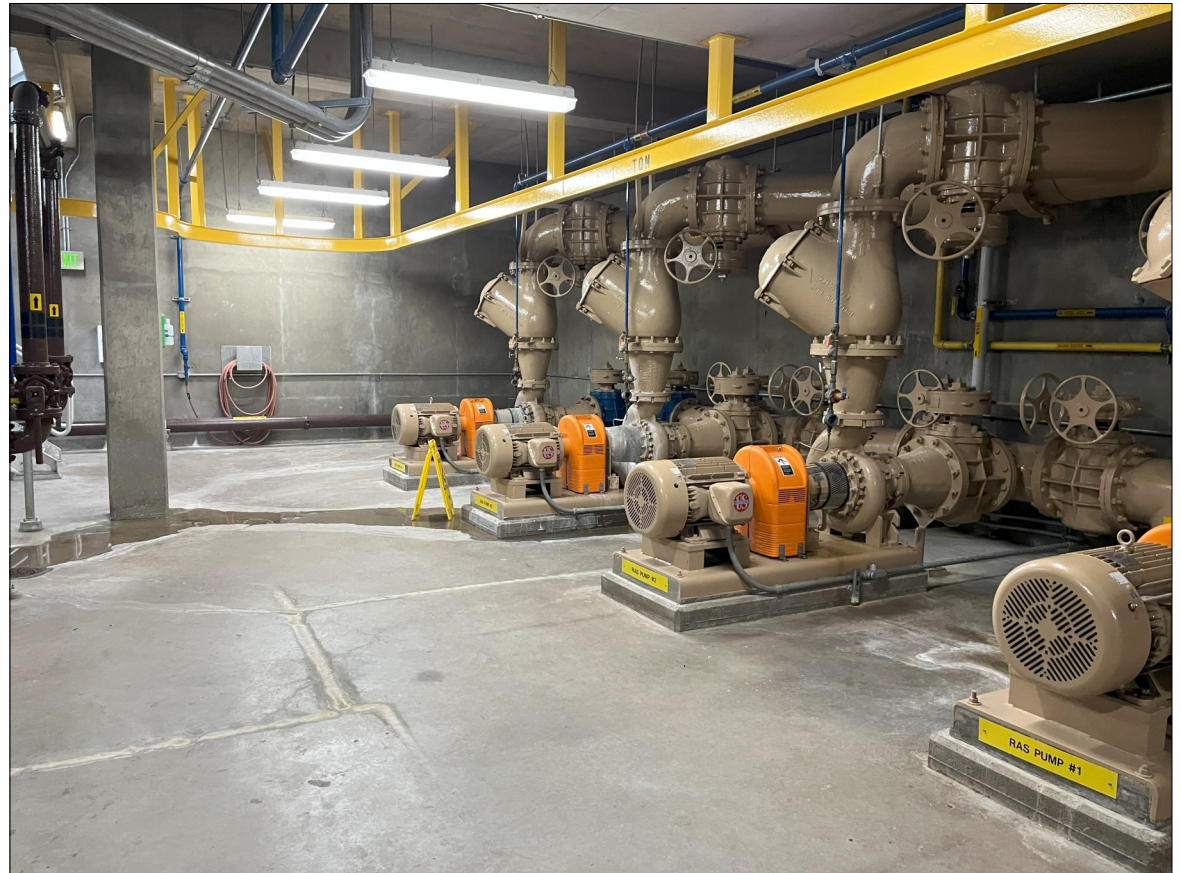
A project to replace failed valves in the return-activated sludge (RAS) pumping system at the Resource Recovery Facility was completed in 2024. The RAS pumps are an important part of the treatment process because they pump beneficial bacteria back to the front of the bioreactors where the hungry bacteria consume nitrogen and phosphorus.
